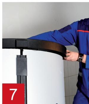
Properly position and attach the lid with the hook strip recesses on top of the thermal insulation.
