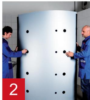
Pull the perforated thermal insulation part with the geomembrane inward over the connections.
