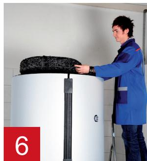
Insert the rondles on top of the tank and position them by pressing them lightly. Caution: To obtain an optimal thermal insulation, there may be no air gap present between the rondle and the thermal insulation.
