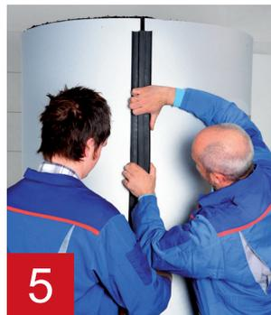
After attaching the cover strip, the thermal insulation can be closed by means of the second hook closure strip. In the case of a three-part thermal insulation, repeat the previous two work processes.
