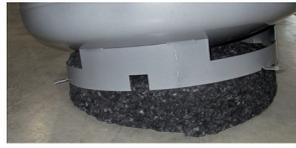
After opening the packaging, properly place the floor insulation and border strip.
